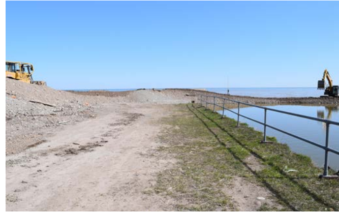
Dredging material from channel
